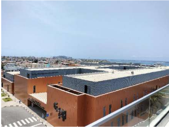
Completion of the Pedalé Hospital Complex Angola
