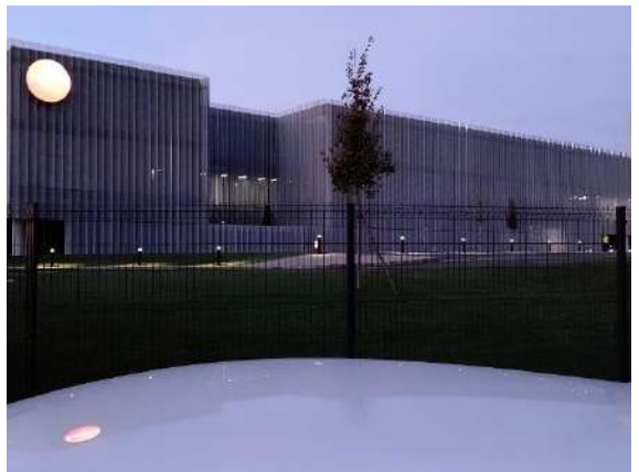
Completion of the Testo Factory Portugal
